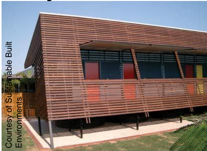
Woodstock House, Melbourne, -Heating climate
